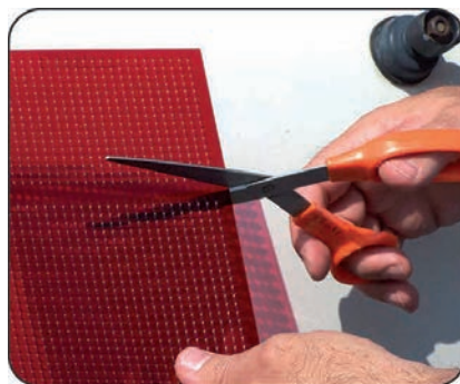
2. Cut the repair panel
